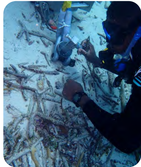
Installation of the first helix anchor at Small Wall
