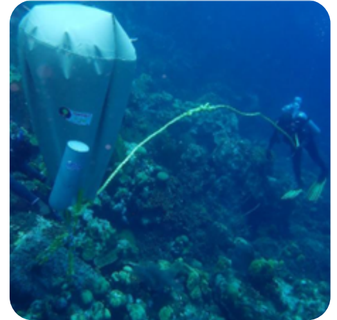
Relocating old mooring block.
